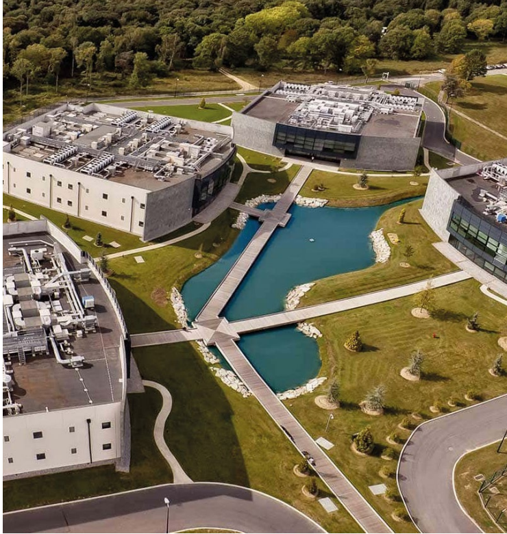
Datacenter, Paris-Saclay © Data4
