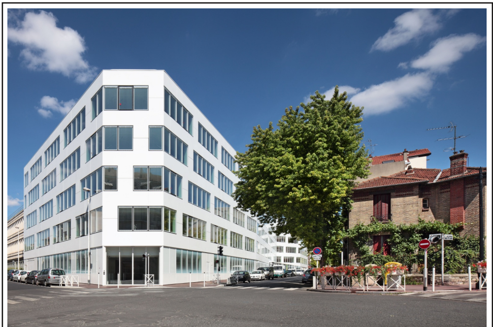
"White", INSEE's new head office building, at 88 Avenue Verdier – Montrouge
